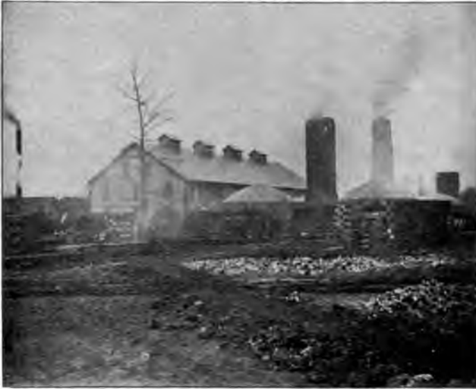
WORKS OF BRAZIL BRICK AND PIPE CO., BRAZIL, IND.
